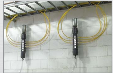
Kaeser Condensate Manifold
