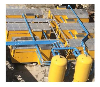
Kaeser's SmartPipe™ is a modular compressed air distribution system that offers lower installation costs and lower long term operating costs. Available in sizes from 1/2"- 6", it's the most versatile compressed air distribution system available.
